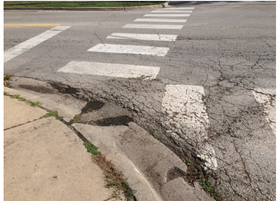
Degradation of crosswalk paint
