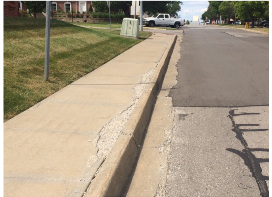
Degradation of sidewalk
