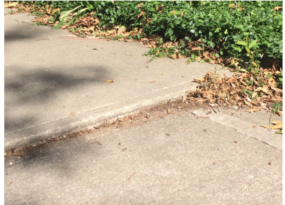
Sudden change in sidewalk elevation
